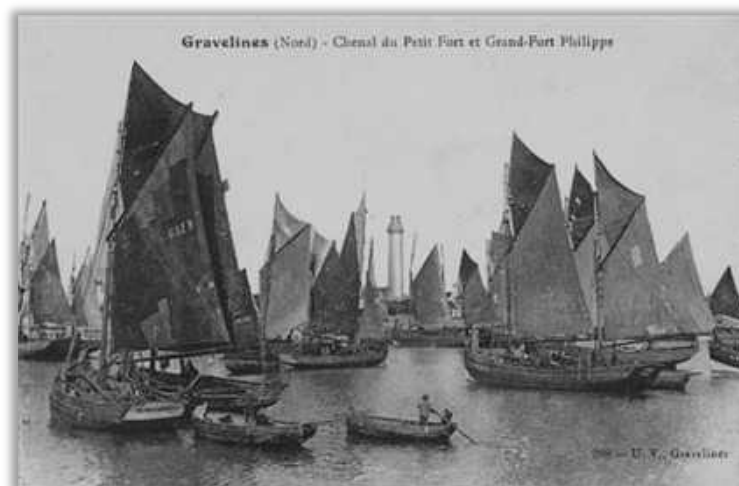
Channel of Petit Fort and Grand-Fort Philippe - Gravelines (North)
